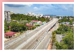
Completed Highway & Flyover From Bayan Lepas To Teluk Kumbar
